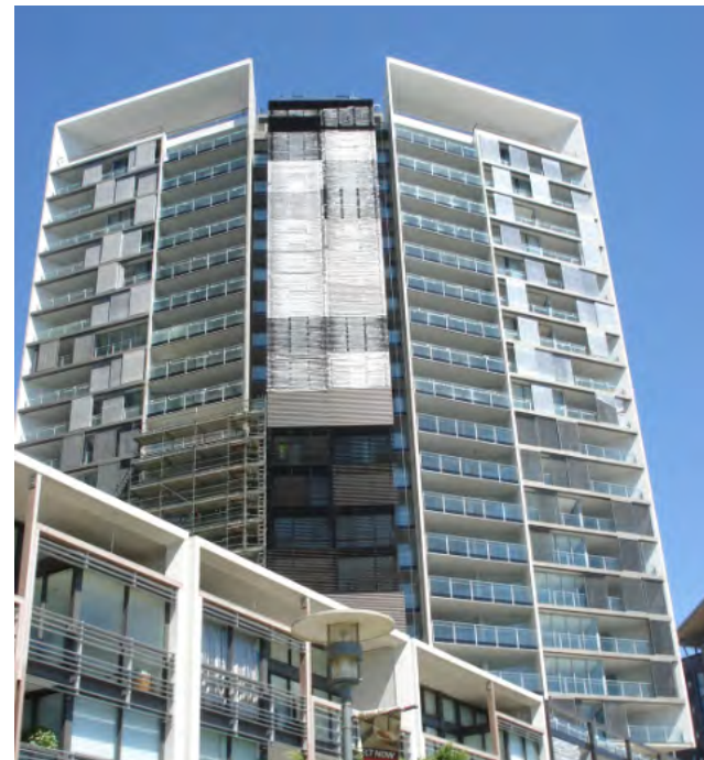
Architectural louver grilles made from extruded aluminum fins
