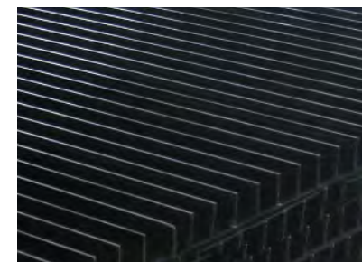
Aluminum rectangular bar grating used as part of an architectural facade designed to have decorative plates attached on the surface.
